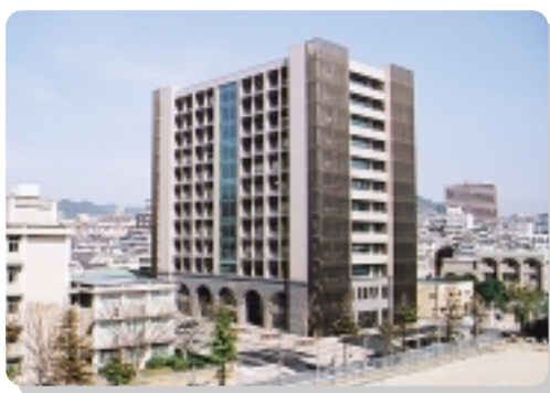
総合教育研究棟 General Education and Research Building
