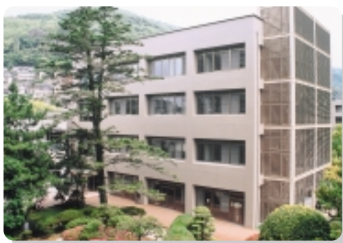
片淵総合教育研究棟 Katafuchi General Education and Research Building
